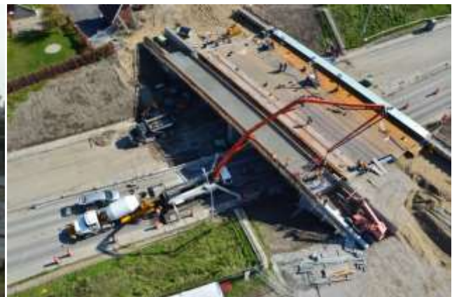
Main St. overpass
